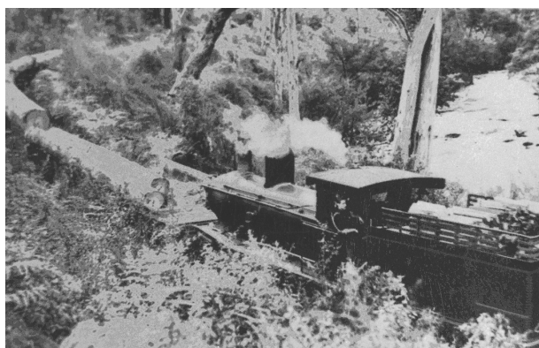
Above: A log train on the 1067mm gauge Goodwood Company's line west of Noojee in Victoria. This is typical of the larger-scale timber tramway systems in Australia, and was based on West Australian practice. (Photo: Rex Jones, author's collection).
