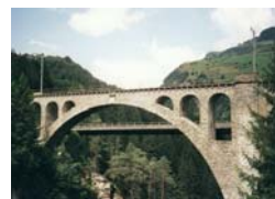
Solis viaduct in Switzerland: Main arc with six "sparing arcs"
